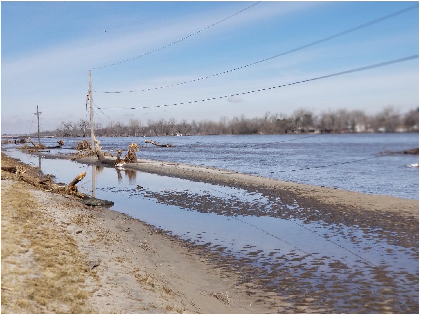
Downed powerlines near the Lincoln wellfield. Photo Credit: Ben Day
