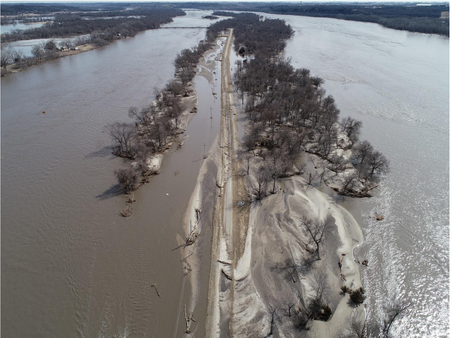
Access road to Lincoln Water System wellfield. Photo Credit: Ben Day
